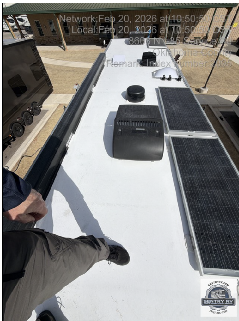
Roof Front to Back
