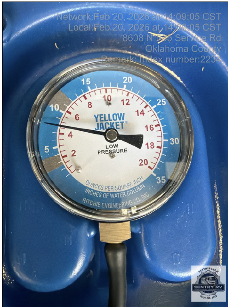
LP Leak Test End
