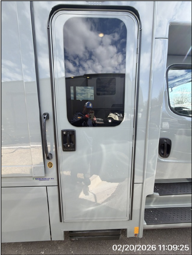
Main Entry Door
