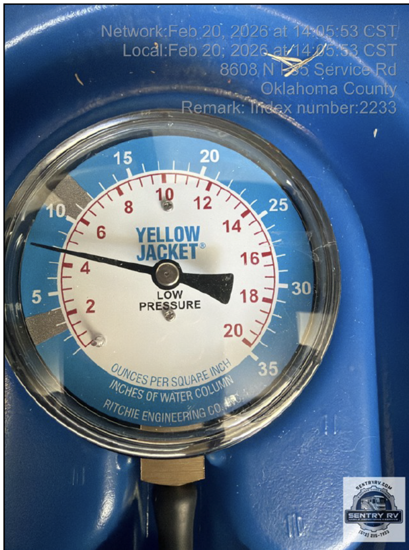
LP Leak Test Start
